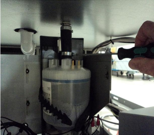
Loosen the 3 nuts to be able to move the unit downwards
