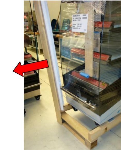
Remove vertical beams and protection on front side
