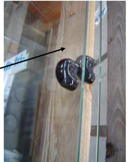
Protective damper between glass Side panel and front door
