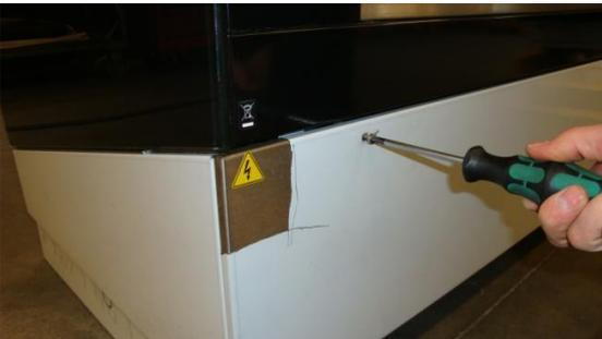
12) Mount the lower skirt on the back side and fasten the screws.
